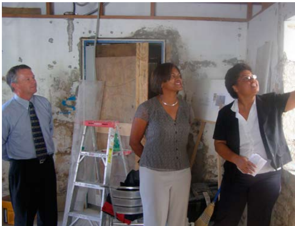
First Caribbean benefactors toured Museum works site in May prior to completion. (From left) Managing Director Tom Crawford and Regional Director for Compliance Anna McLean with the Museum's Acting Director Debra Barnes-Tabora (far right).
